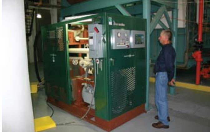
Gulf Coast Green Energy Technical Manager Chris VandenBergh checks out his company’s “Green Machine” Waste Heat Generator in operation in a boiler room at Southern Methodist University in Dallas. The stand-alone unit captures waste heat from almost any geothermal or industrial source to generate fuel-free, emission-free electricity.
